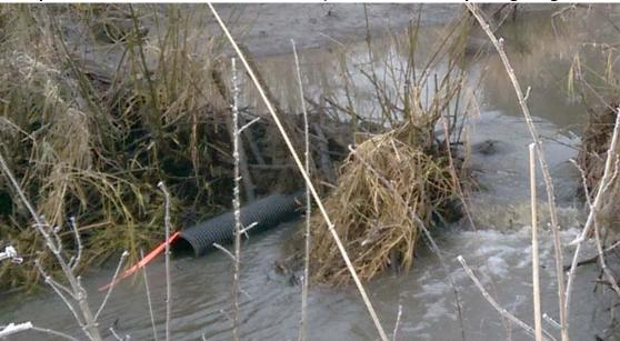
Example of a flow device installed ina dam. (The end is noted by orange flag in water)
