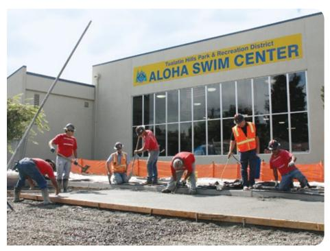
Workers install a new pervious concrete parking lot and sidewalk at the Aloha Swim Center, one of many sustainable approaches to new projects. Permeable surfaces reduce and filter the stormwater runoff entering local streams.
